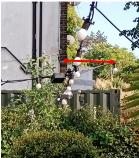
Figure 1 Container sits forward of main elevation of neighbour
